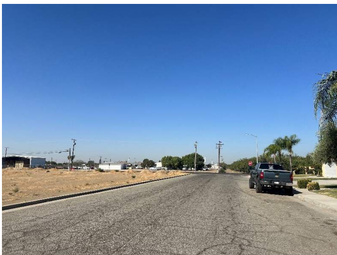
Street View Looking West along Redwood Dr.
