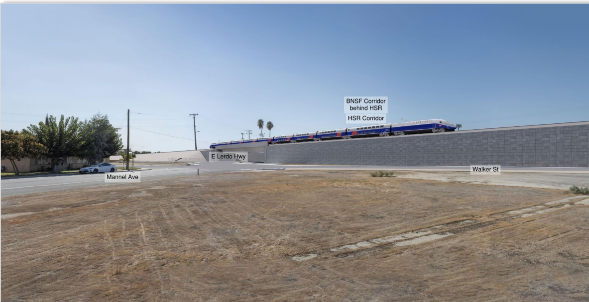
Retained Fill Variation: E Lerdo Hwy Underpass (on Mannel Ave looking southeast)
