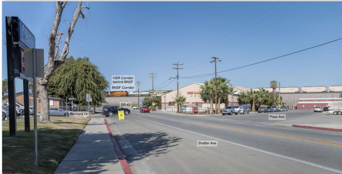
Retained Fill Variation: Shafter Ave Underpass (on Shafter Ave looking north)
