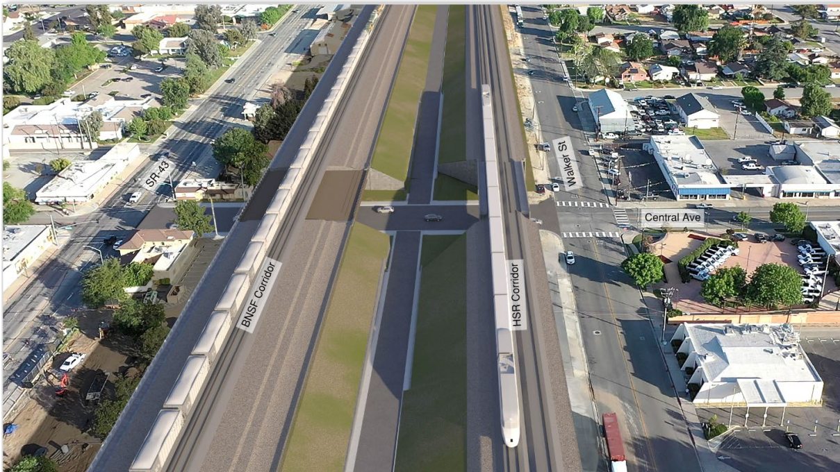
Retained Fill Variation: Central Ave Underpass (aerial view looking northwest)
