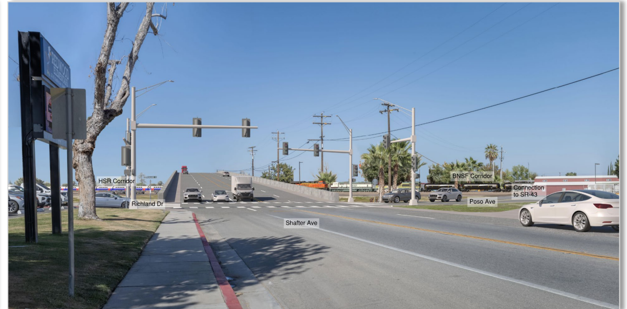
Grade Separated Variation: Shafter Ave S-1 Overpass (on Shafter Ave looking north)
