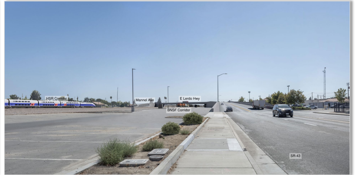
Grade Separated Variation: E Lerdo Hwy L-2 Overpass (on SR 43 looking southeast)
