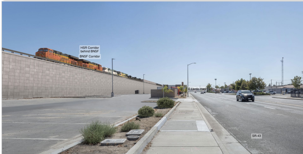
Retained Fill Variation: E Lerdo Hwy Underpass (on SR 43 looking southeast)
