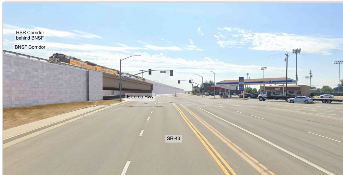
Retained Fill Variation: E Lerdo Hwy Underpass (on SR 43 looking southeast)
