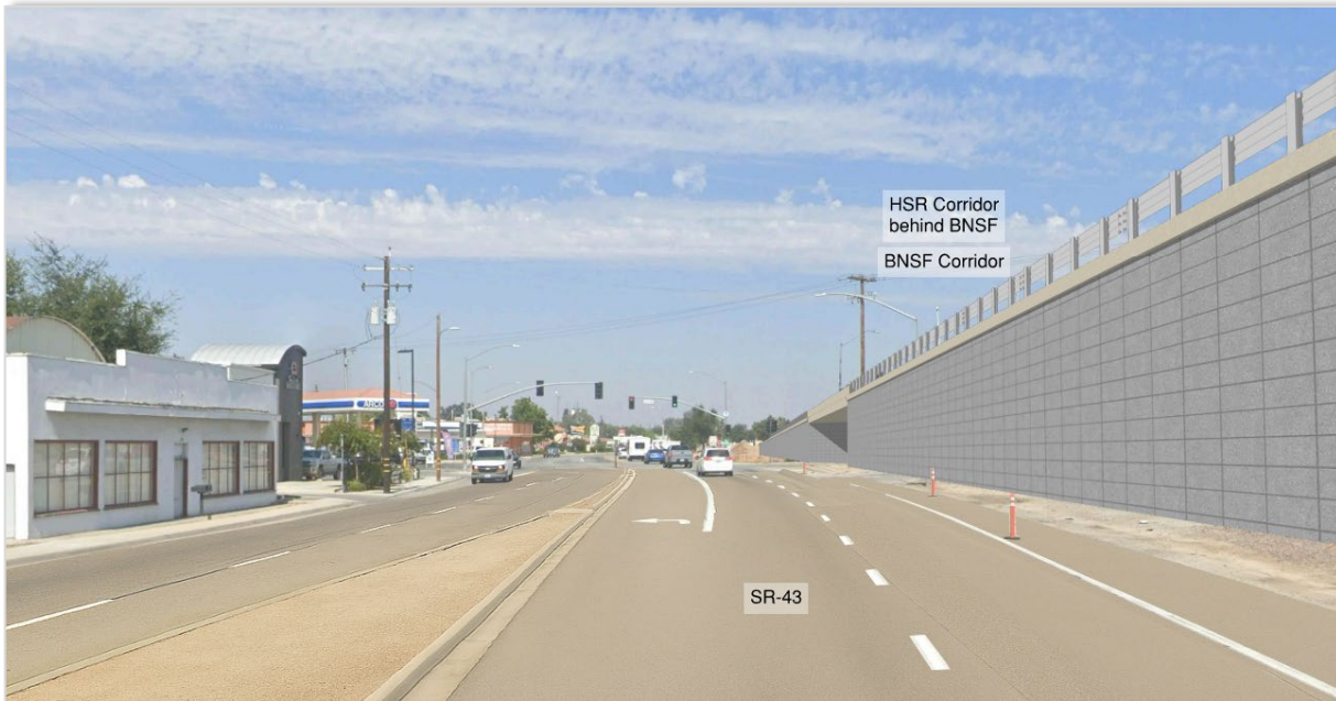
Retained Fill Variation: E Lerdo Hwy Underpass (on SR 43 looking northwest)
