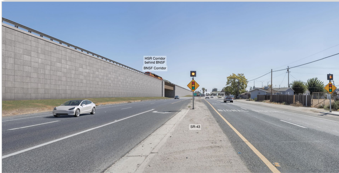
Retained Fill Variation: Shafter Ave Underpass (on SR 43 looking southeast)
