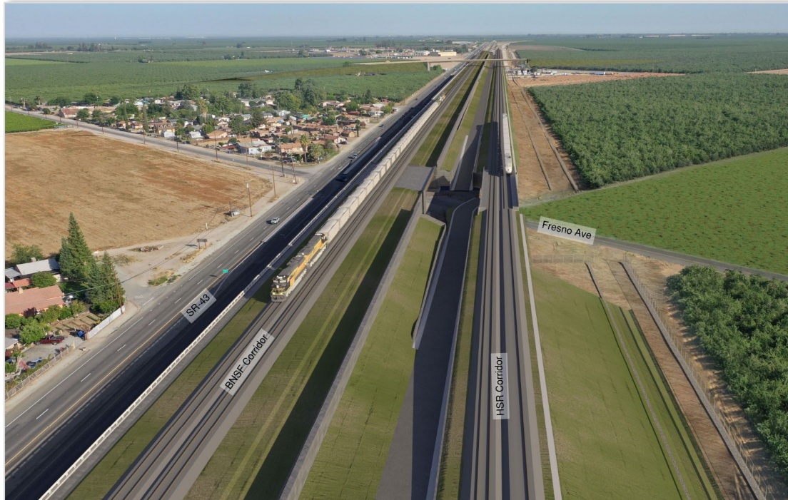
Retained Fill Variation: Fresno Ave Underpass (aerial view looking northwest)
