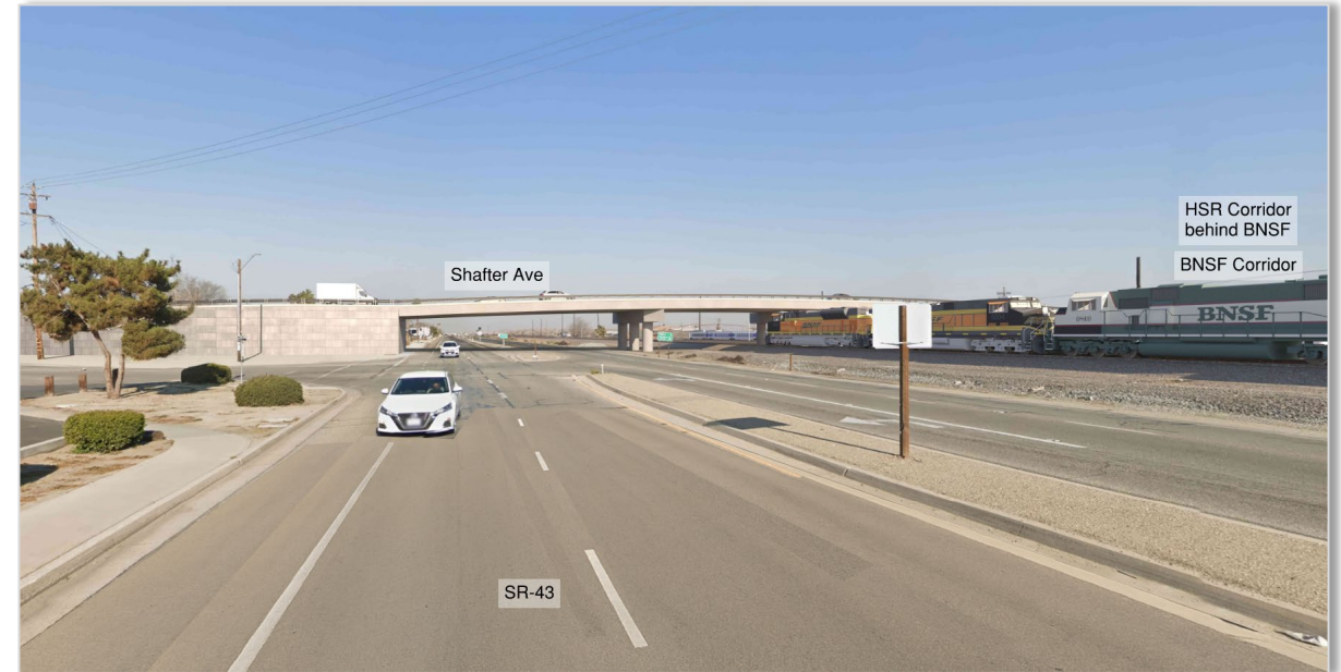
Grade Separated Variation: Shafter Ave S-2 Overpass (on SR 43 looking northwest)
