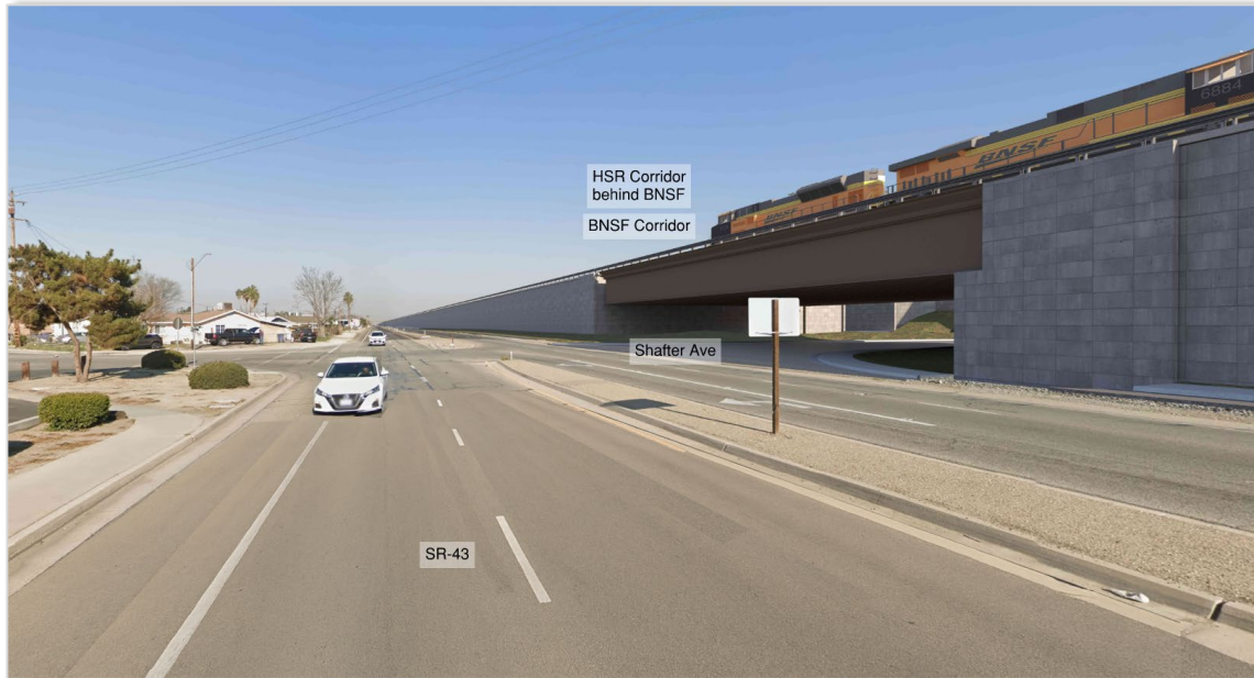
Retained Fill Variation: Shafter Ave Underpass (on SR 43 looking northwest)
