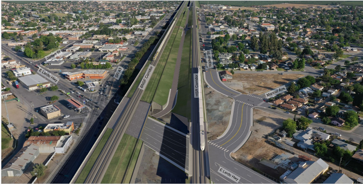
Retained Fill Variation: E Lerdo Hwy Underpass (aerial view looking northwest)
