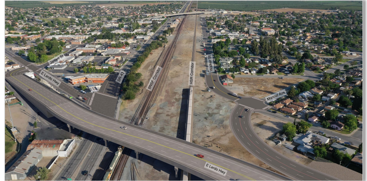
Grade Separated Variation: E Lerdo Hwy L-1 Overpass (aerial view looking northwest)
