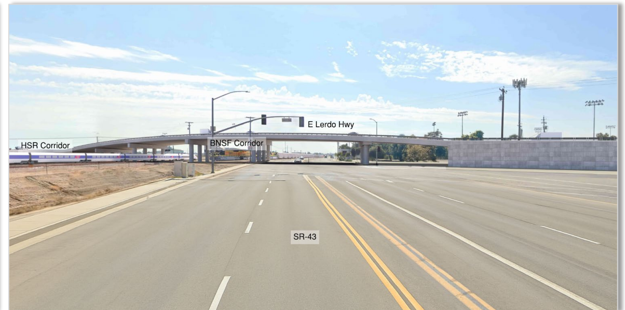
Grade Separated Variation: E Lerdo Hwy L-1 Overpass (on SR 43 looking southeast)
