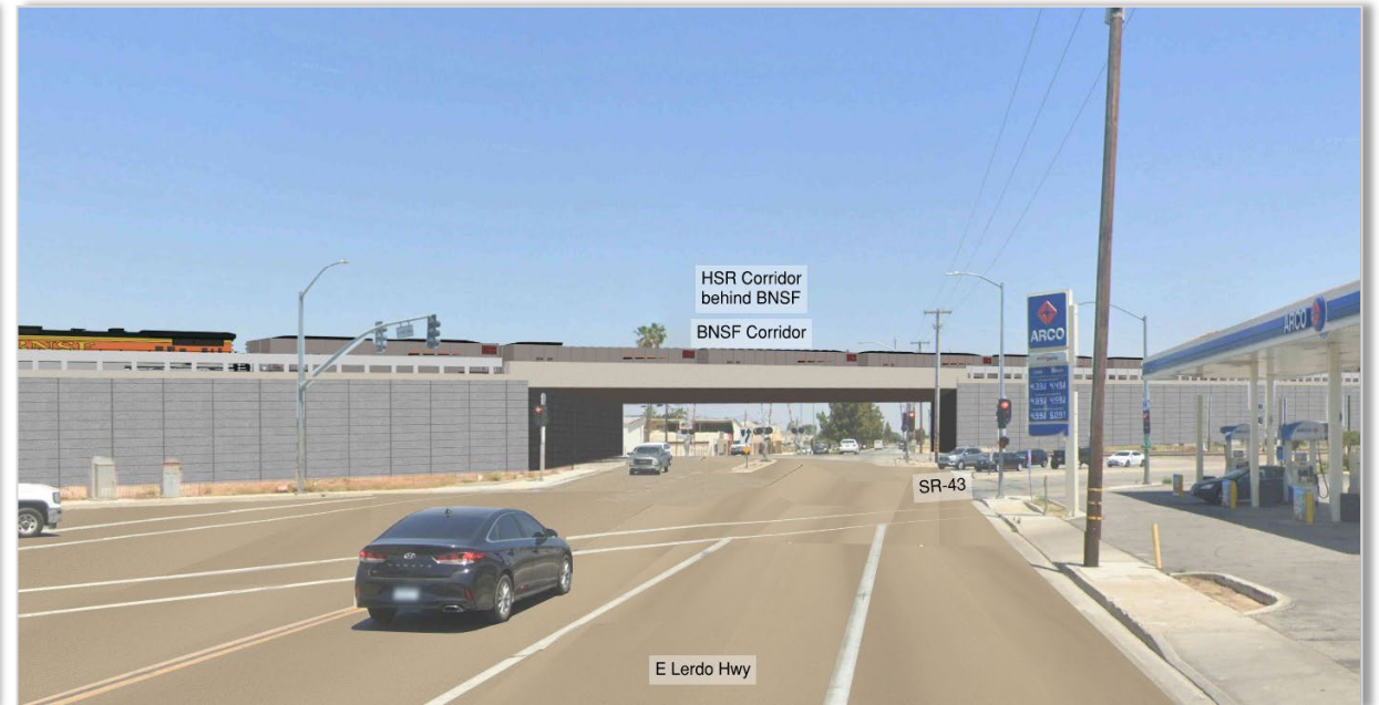
Retained Fill Variation: E Lerdo Hwy Underpass (on Lerdo Hwy looking east)
