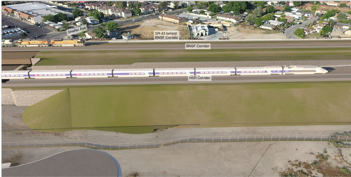
Retained Fill Variation: Shafter Ave Underpass (aerial view looking southwest)
